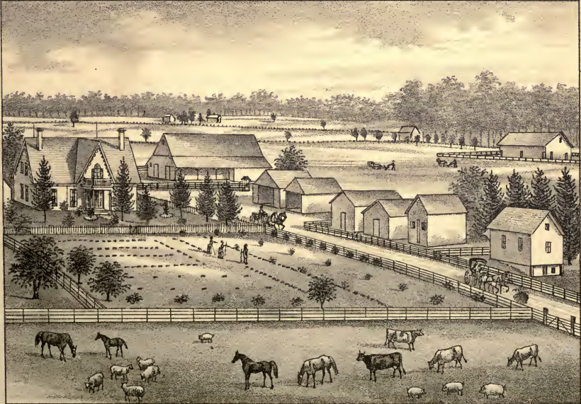
RESIDENCE & FARM OF DAVID ADAMS, SEC. 21, T. 1, R. 12, WABASH PRECINCT, WABASH CO. ILL.
